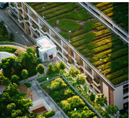
Figure 8.18: Green Roof on Podium
